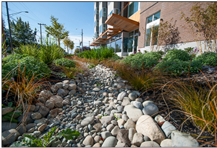
A bioswale along South McClellan Street filters rainwater from the alley and street.
